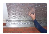
4. This picture shows the sheeting then going over the top edge and butting up ready for fixing in place. Sheeting can be started from the centre of the room or the cornice edge.
