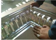
5. Picture shows both cornices coming together, just as they will be when installed. Minor trimming may be required to perfect the joint.
