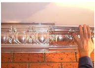
7. Install the next length of cornice into the mounting strip, overlapping the previous cornice. Some paintable no-more gaps may be smoothed over the joint to help it to appear seamless.
